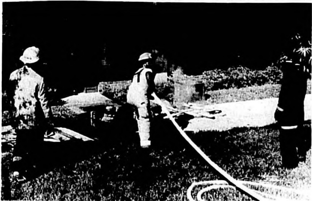
Sanford and Altamonte Springs firefighters hose down smoldering books and other items pulled from the SCC vocational education building.
