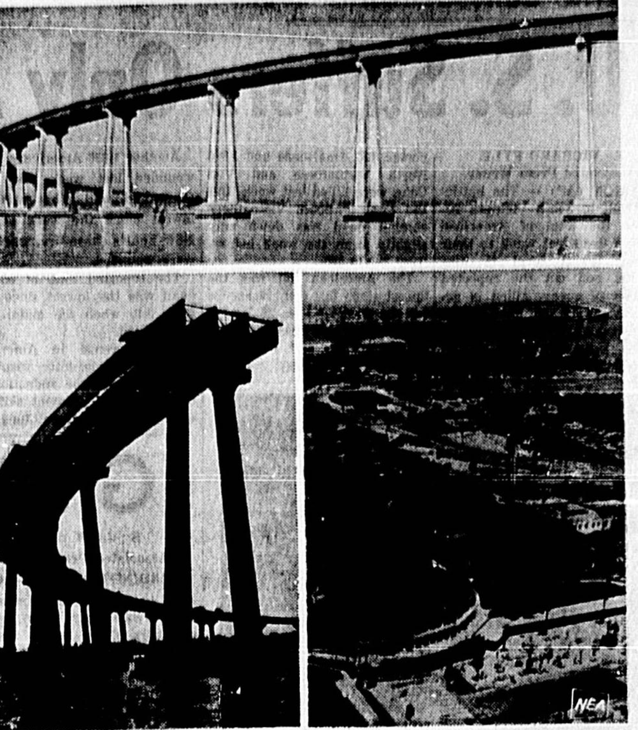
SPANNING SAN DIEGO BAY, this new $28-million bridge links the California cities of Coronado and San Diego. Reportedly one of the most beautiful bridges in the world, a team of specialists in aesthetic design participated in the plan to make sure every advantage of natural environment was considered. Dramatic shot at bottom left shows curved section in construction last year. Bottom right photo was taken from Coronado side after bridge's completion.
