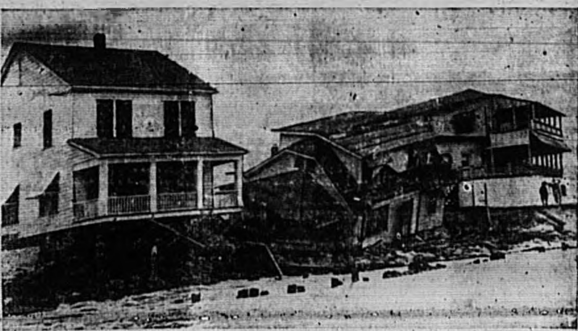
THESE TWO HOUSES WERE WRECKED at Smyrna Beach, Fla., after a flash storm at sea off the northeastern coast of Florida caused excessive high tides. Numerous homes and buildings along the State's beach-fronts were damaged. In the area near Jacksonville damage was estimated at about $300,000. (International)
