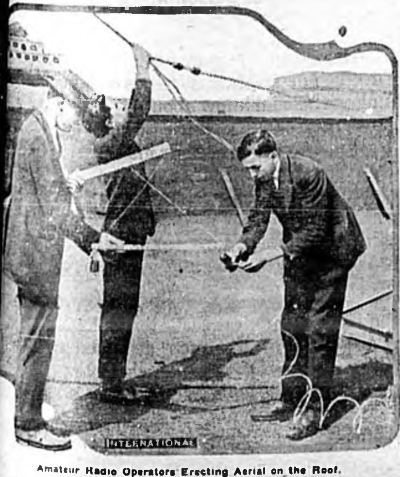
Amateur Radio Operators Erecting Aerial on the Roof.
