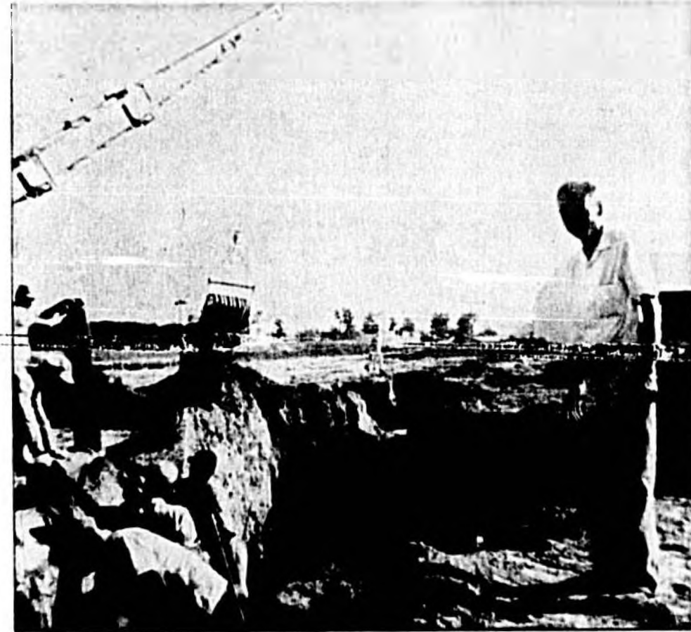
CASSELBERRY UTILITY CO. crews began last week laying water and sewer lines to the newly annexed Seminole Plaza Shopping Center located at the junction of SR 436 and Hwy. 17-92. Company Superintendent Paul Bates, right, is in charge of the work. (Herald Photo)
