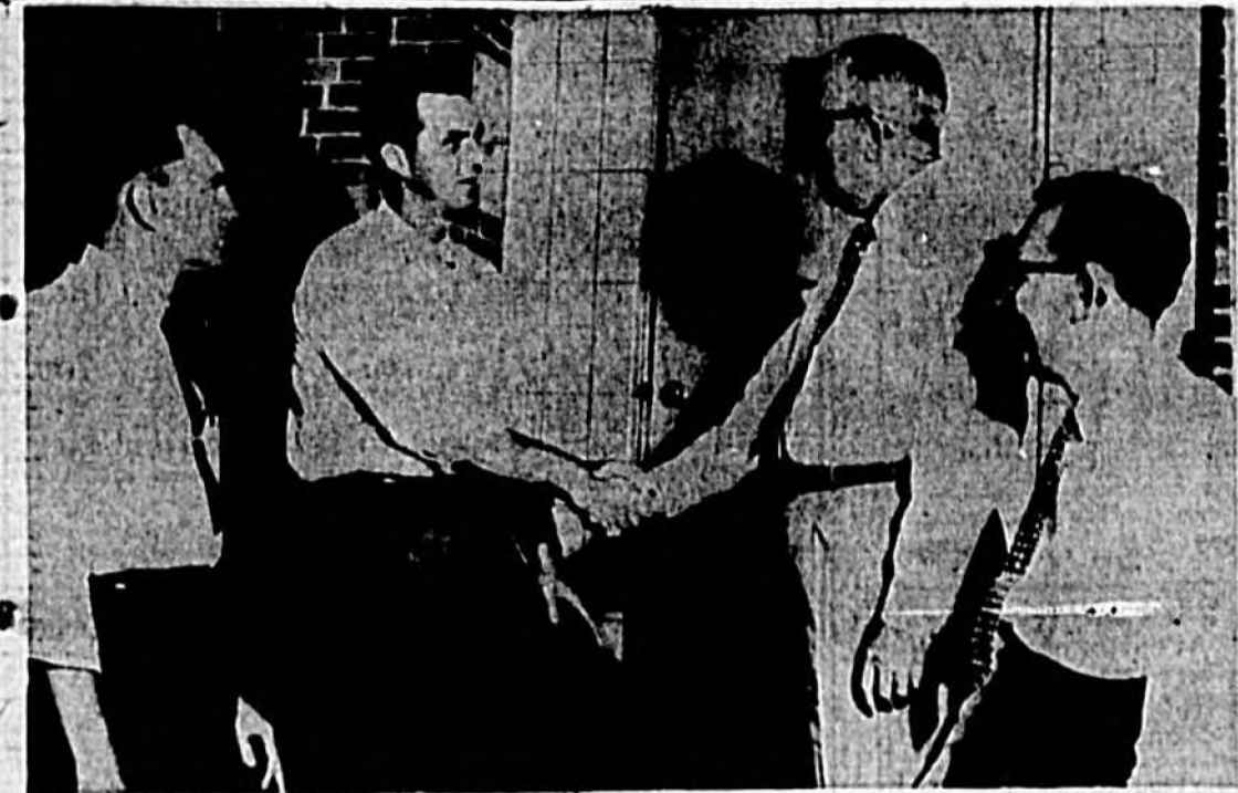
WESTERN ELECTRIC SUPERVISORS who will install new dial equipment and switchboards in the Southern Bell Telephone and Telegraph Co. building on Laurel Ave. and Ninth St. (Left to right) Carl Jones, J. E. Kuehn, Earl Turner, local manager and Gordon Rothermel, Sanford-Deland Group Manager. (Photo by Jameson)
