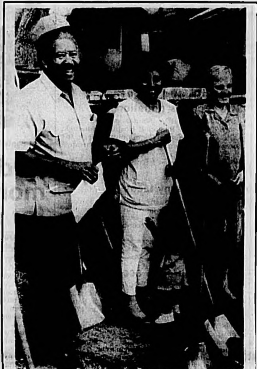
Another affordable house GoldenRule Housing and Community Development broke ground Friday for the third in the series of five affordable housing units. The home is being built in the 1800 block of W. 5th Street Sanford. Shown during the ceremony, left to right, Willie King, President of GoldenRule, Delores Felton, buyer of the new home, her granddaughter Sharkyrie Balton, and Sanford Mayor Bettye Smith. The home is expected to be completed and ready for occupancy by the Feltons within 60 days.
