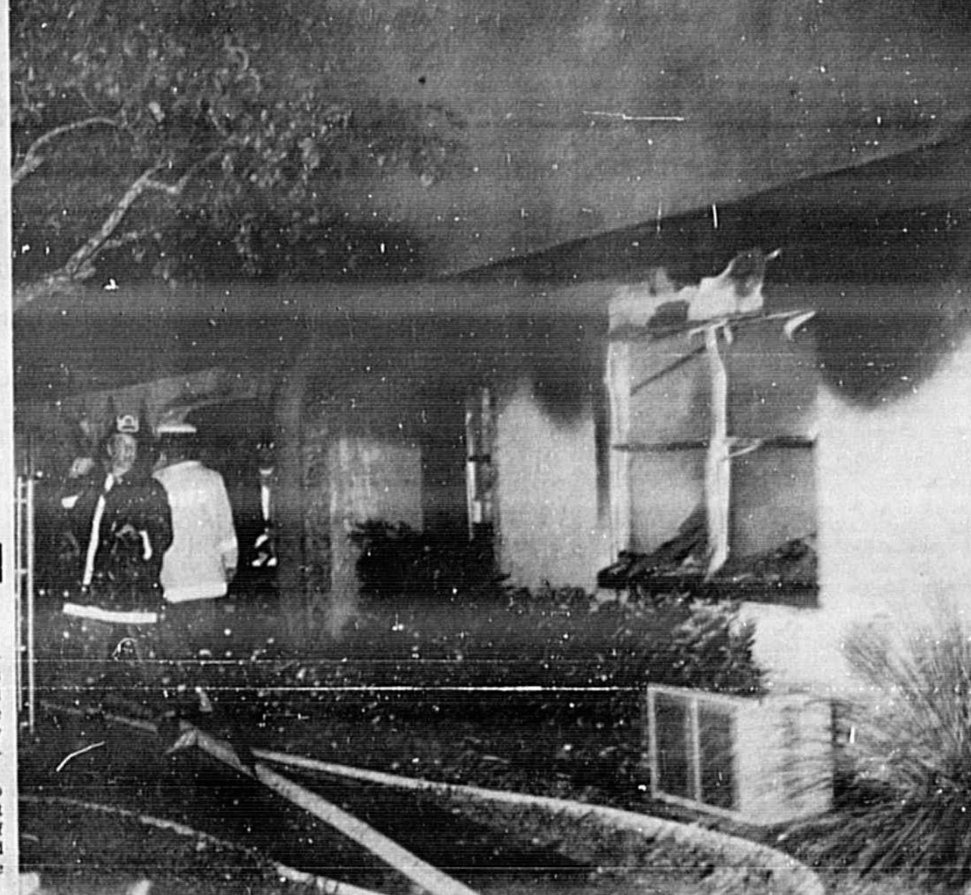
APARTMENT GUTTED BY FIRE Fire from an undetermined origin early today caused an estimated $30,000 loss to a South Seminole apartment; additional furnishings loss was placed at $5,000. juries in the blaze that destroyed unit 65 of Sorrento Apartments, located at 2400 Howell Branch Road in Casselberry. (Additional photo page 2A.)
