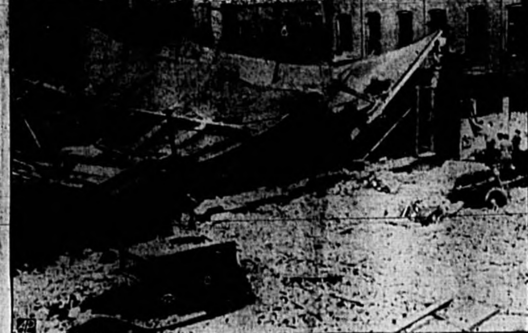
At least one person was killed and 40 others were injured in a terrific explosion that demolished a brick factory at Paterson, N. J. Houses were jarred for blocks around. The blast was believed to have originated in a gas oven. The wreckage of the building is shown shortly after the explosion. Note the automobiles partially buried under debris.
