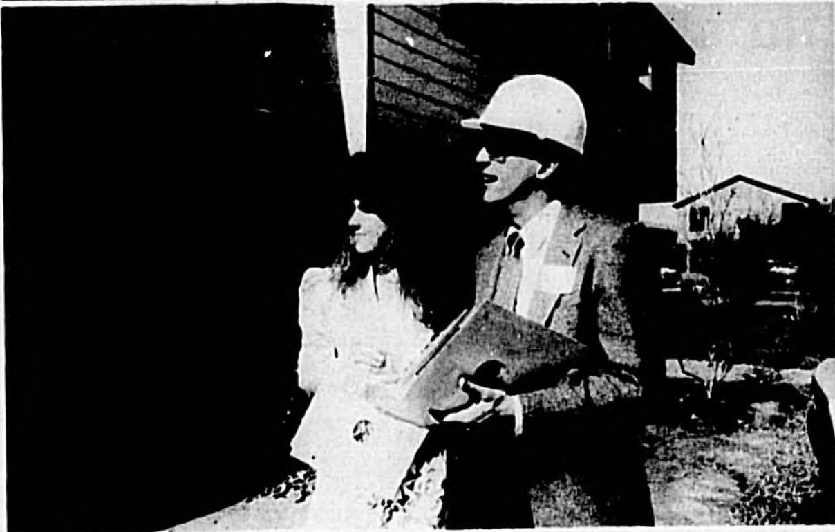
First Union Consumer associate Susan Casey and Commercial lender Steve Allman were among local guests touring the Cedar Creek Apartments affordable housing units, still under construction.
