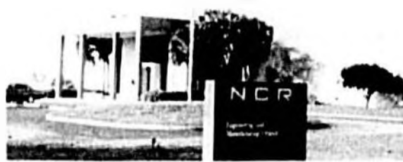
The NCR plant in Lake Mary this morning
