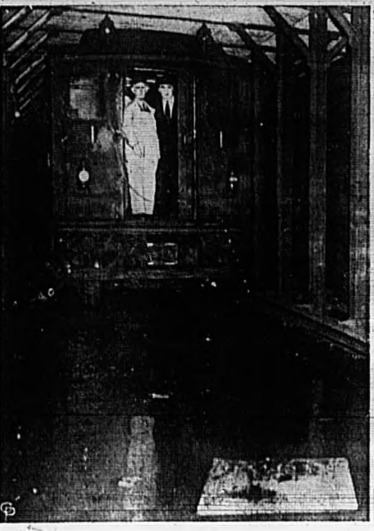
A BREAK IN A 36-INCH water main on New York's West Side brings a subway train to a halt on the IRT line at 80th Street and Broadway. Nine thousand passengers were trapped for a short time when water poured into the tunnel. Service was suspended 5 hours. (International)
