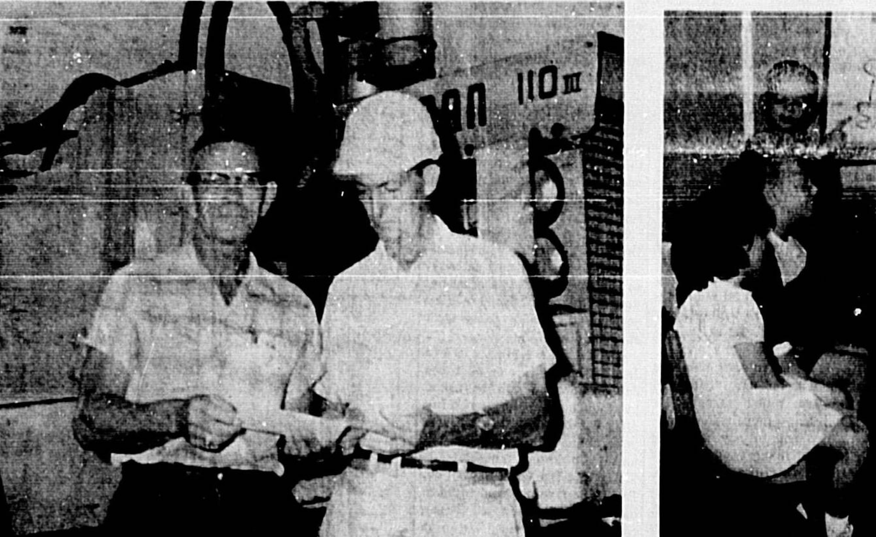
WORK began Monday morning on preparing the site for the million dollar K-Mart Shopping Center on Highway 17-92 in Fern Park south of the Jai Alai Fronton. Target date for the opening of the K-Mart department store and a food store is April 1. Other retail stores will be added. Tim Hartnett (left), superintendent for Hannon South Construction, contractors, gives instructions to Eddie Parker, earth mover. (Jane Casselberry Photo)
