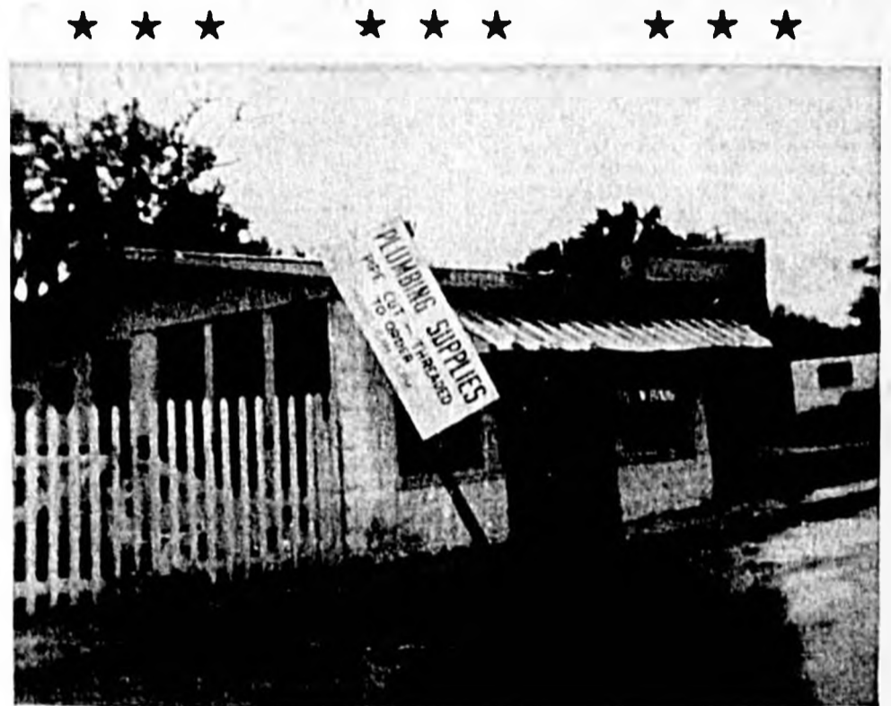
HURRICANE FORCE WINDS ripped off the sign and part of the roof at George Reek and Son Plumbing on E. Lake Ave. in Longwood during this morning's wind and rain storm onslaught which hit the entire South Seminole area. Damages were estimated at some $200 to the building. (Herald Photo)
