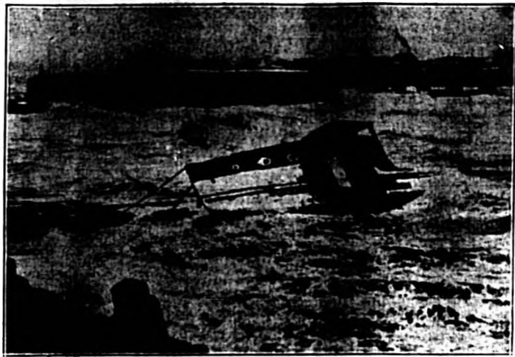
Damage estimated at several million dollars was done by a terrific gale that pounded the eastern seaboard from New England to North Carolina. This picture, made at the peak of the storm swept Long Island, New York, shows the wreckage of a yacht and docks undergoing a severe battering. (AP Associated Press Photo)
