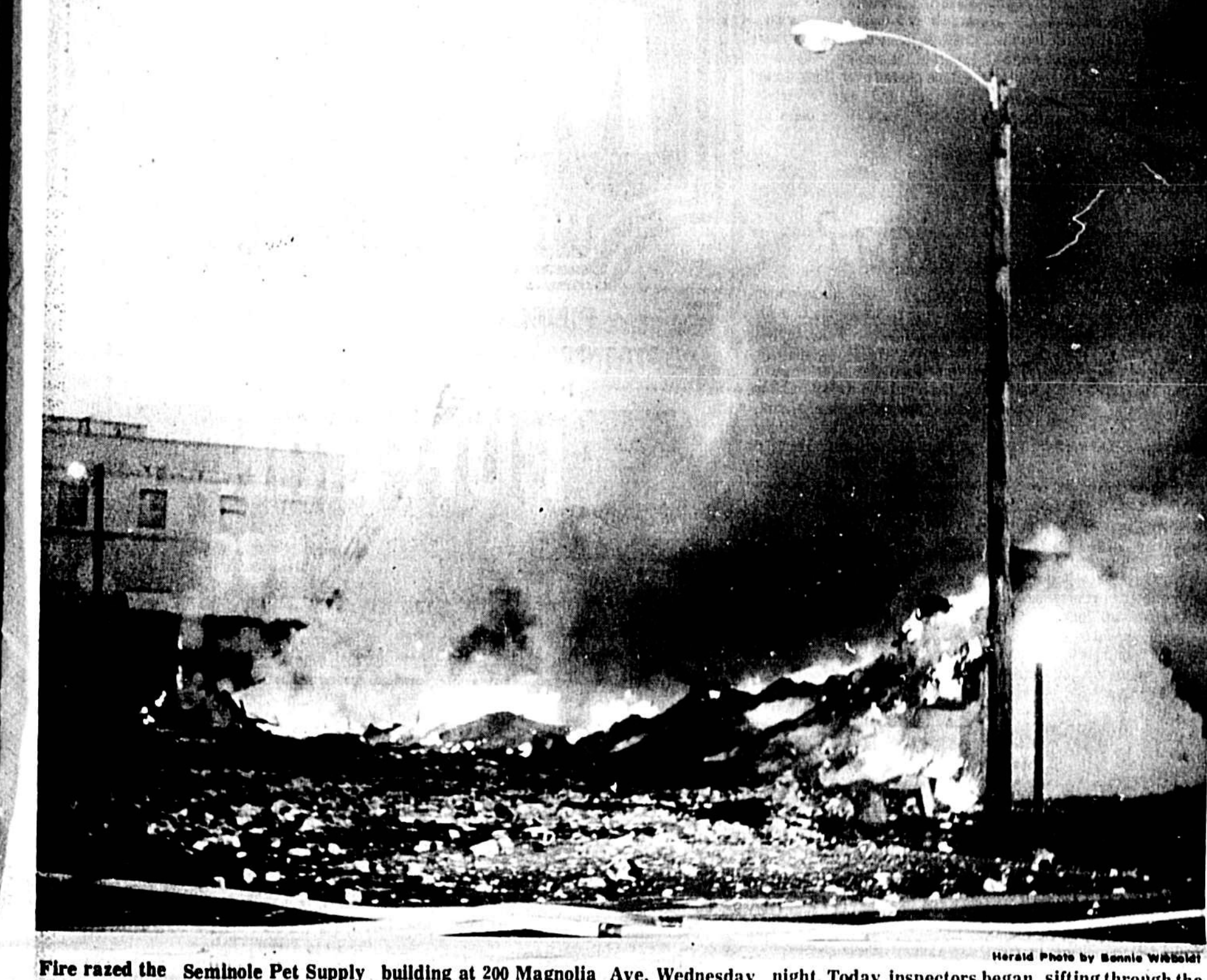
Fire razed the Seminole Pet Supply building at 200 Magnolia Ave. Wednesday night. Today inspectors began sifting through the charred rubble for clues as to the cause of the blaze.
