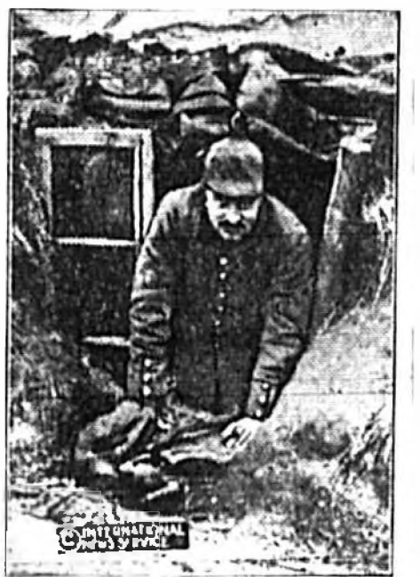
Underground Houses in the German Trenches in Poland.
