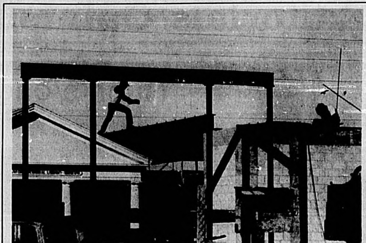
Progress on museum
