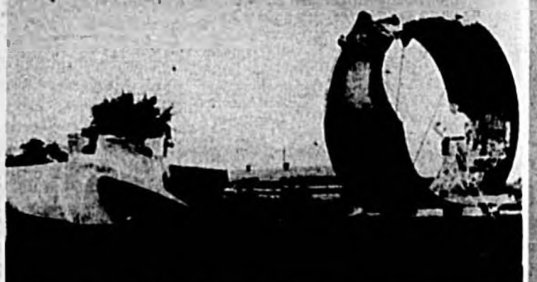
A CASTING for one of the six pumps (right) and one of the 17,000 pound manganese bronze propellers almost dwarf flat car on which they were delivered to Twenty Mile Bend.
