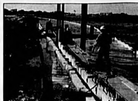
Below: Crews set some of the first seawall panels on the Sanford Riverwalk near Mellonville Avenue. Above: The final seawall panel for the Riverwalk project is installed at Memorial Park.
