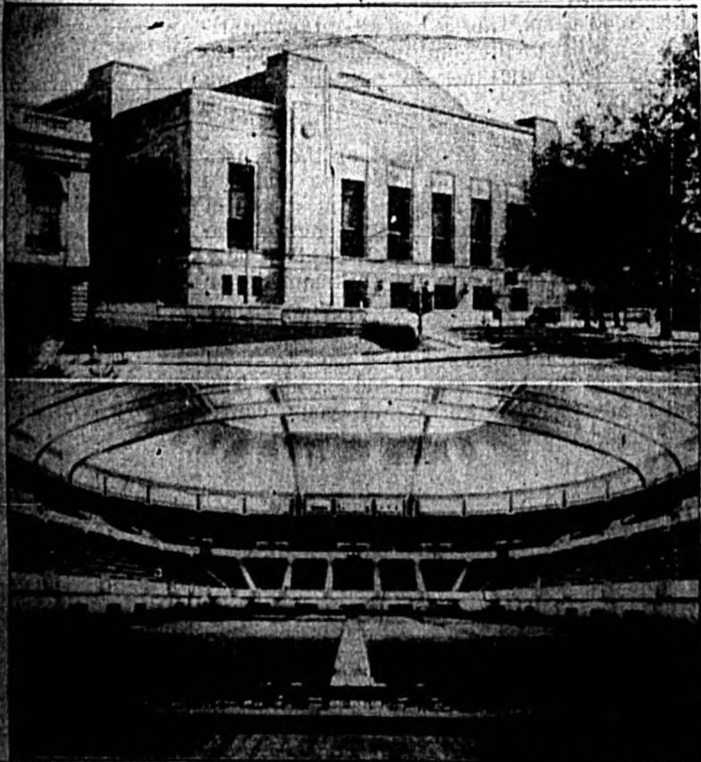
Exterior and interior views of the Municipal Auditorium in Philadelphia where the delegates to the Democratic National Convention will meet June 23. The Democratic Executive Committee meeting at Washington selected Philadelphia as the convention city after eager citizens put up a cost $200,000, offered facilities free and promised "to ring anew the Liberty Bell." (Associated Press Photos)
