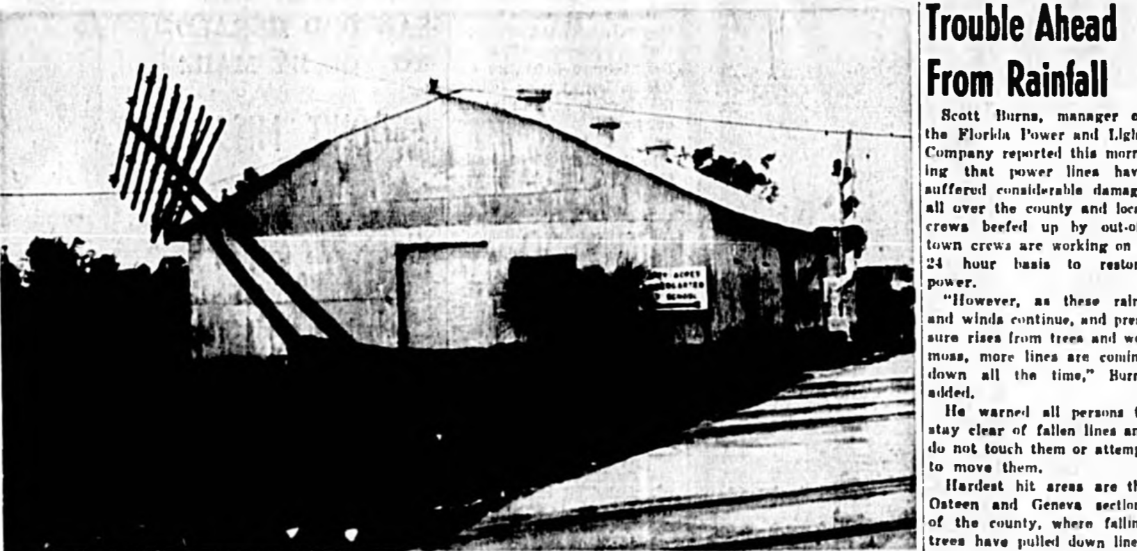
WIND TOPPLES WIRES AGAINST BUILDING
