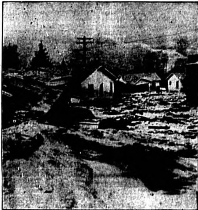
This is the second time this year that residents of Montrose, Calif., have had their homes wrecked by flood waters rushing down from mountain canyons. This picture shows what the flood did to the town. Montrose was struck by a flood of similar size on New Year's day. (Associated Press Photo)
