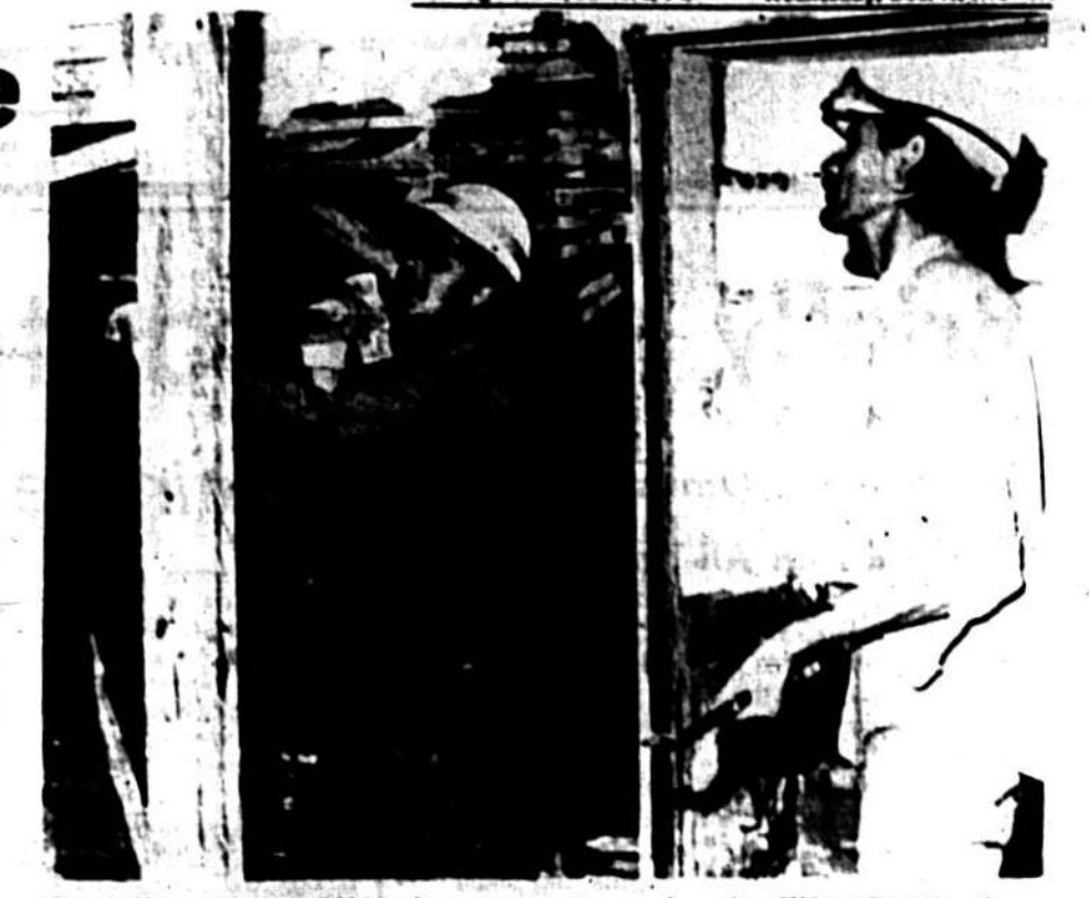
Ray Tulman (left) and Ed Rehn, construction workers for Clifton Construction, do their thing in Welaka building.
