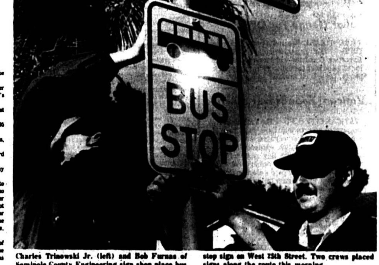
Charles Trinoski Jr. (left) and Bob Furnas of Seminole County Engineering sign shop place bus stop sign on West 23th Street. Two crews placed signs along the route this morning.
