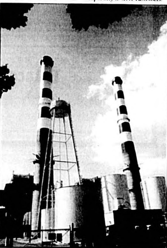
Florida Power & Light is preparing to repower the Sanford Power Plant, a move which will create about 950 jobs.
