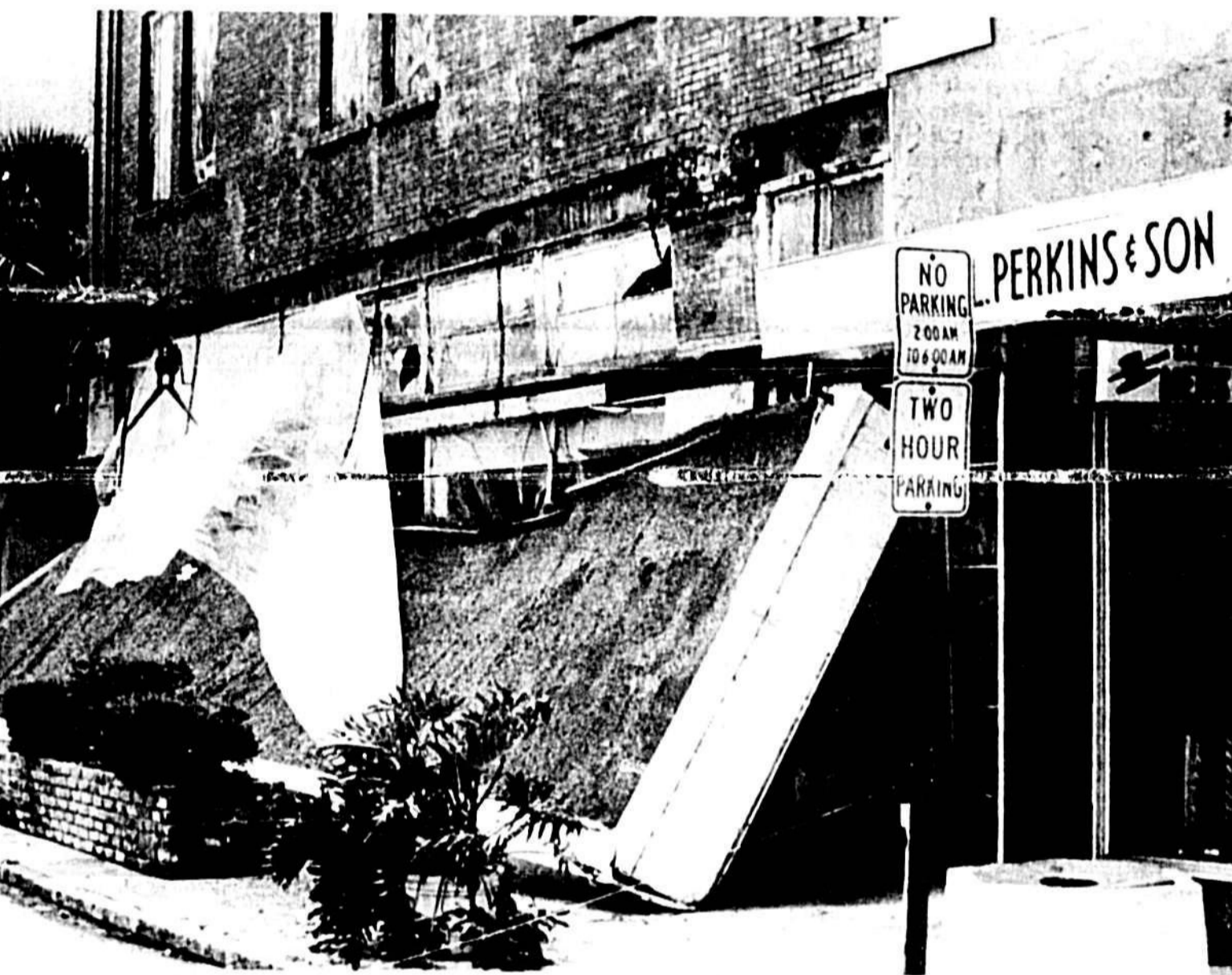
THE CANOPY CAME DOWN Four workers escaped injury Thursday when the canopy they were standing on above the first floor of Garrett's Department Store at 200 E. First St. in Sanford collapsed. Portions of the canopy smashed the front window of the building. Total damage was estimated at $18,000. Investigators said the collapse of the canopy occurred when four metal support cables broke.
