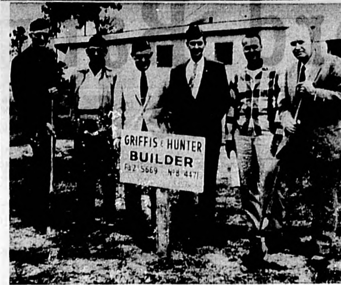
LEGION BREAKS GROUND — Legionnaires in Sanford today broke ground for the new fair building, which will adjoin the new home on Highway 17-92. Left to right, J. G. (Slim) Galloway, J. D. Cordell, George Mayberry, Bob Mahan, John Griffis, contractor, and Joel Field, commander. (Bergstrom Photo)
