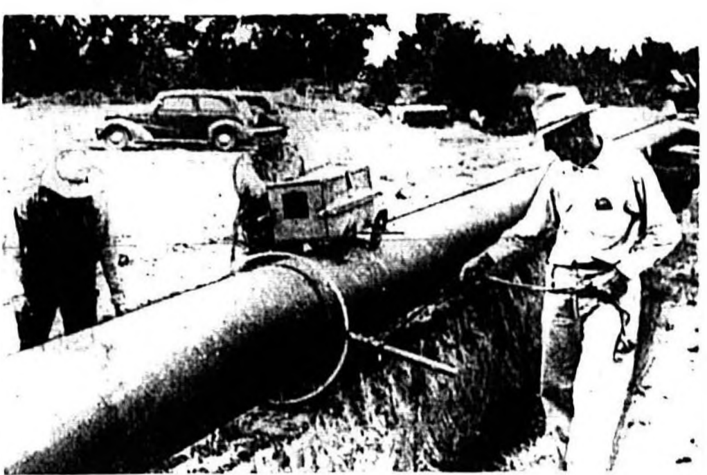
Workers laying the pipeline for the oil pipeline.
