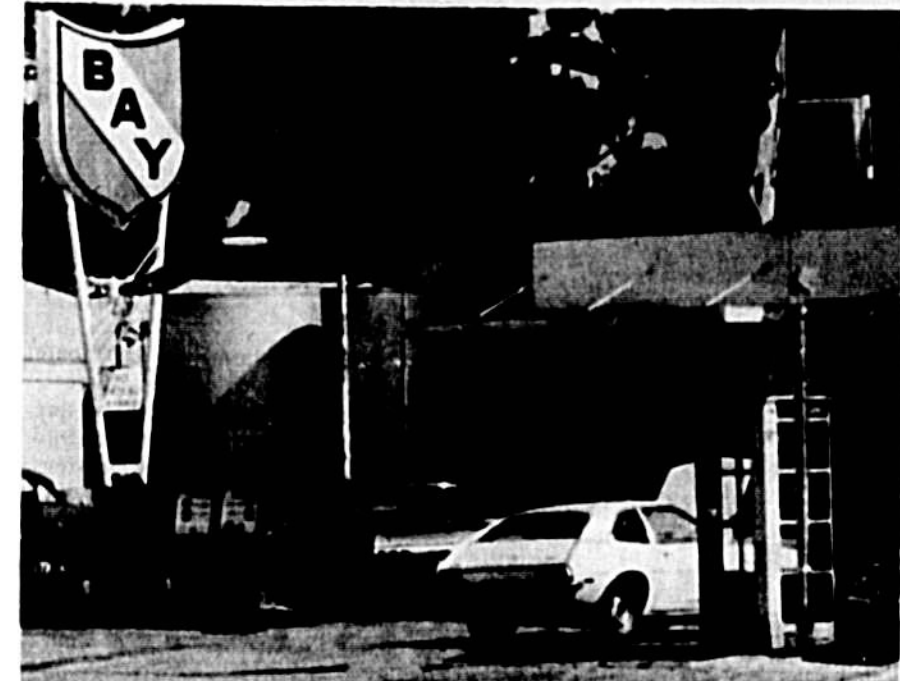
GAS STATION. FUEL STORAGE TANKS SIT ATOP TRAPPED GAS
