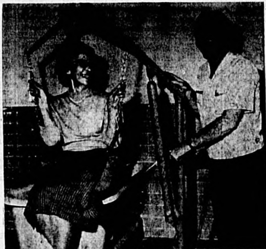
Mr. Halback, President of Wall Plumbing and Heating, and Mrs. Graham, Sr. demonstrate the hydraulic lift used to lift patients in and out of the institutional tub in the special bathroom for patients unable to bathe themselves.
