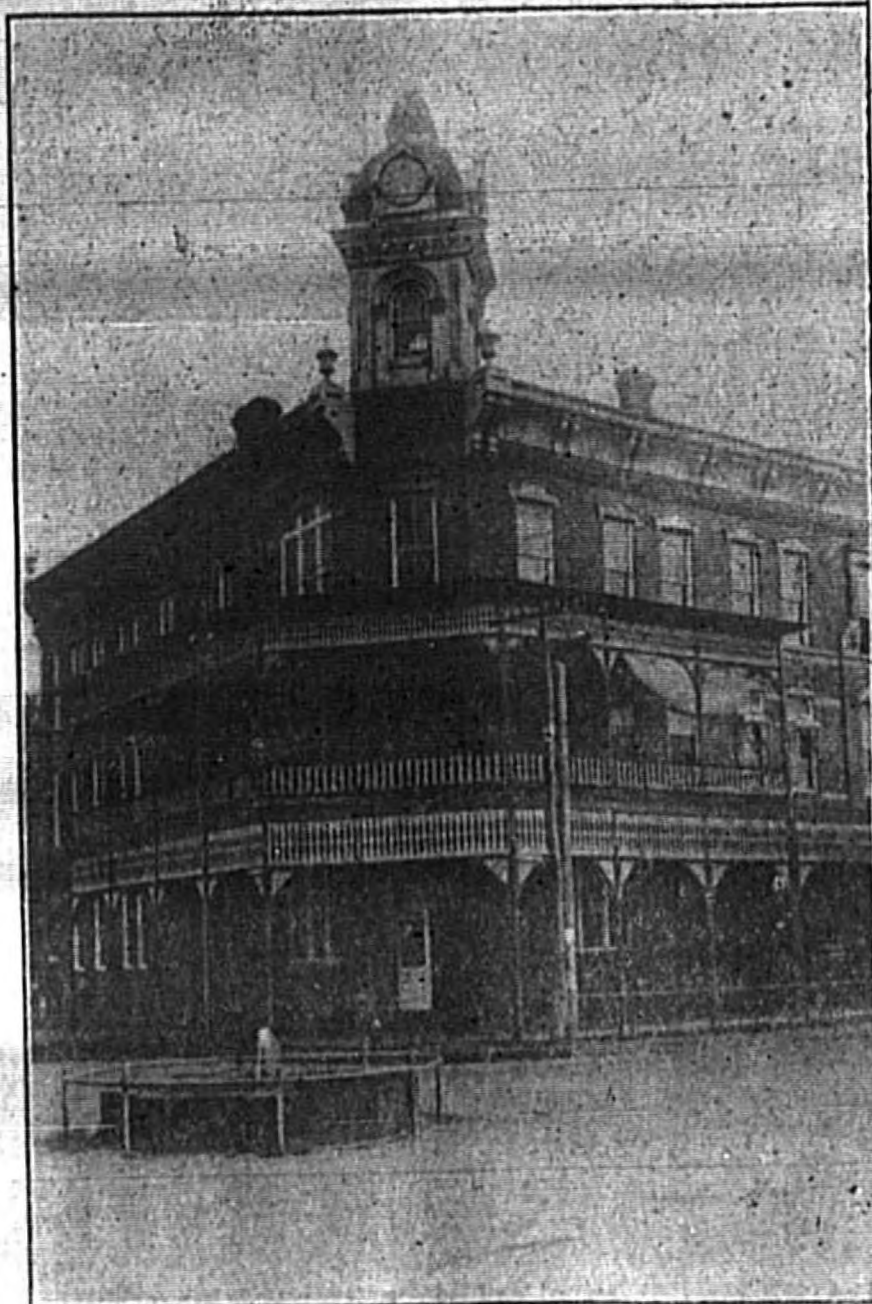
SEMINOLE BANK BUILDING
