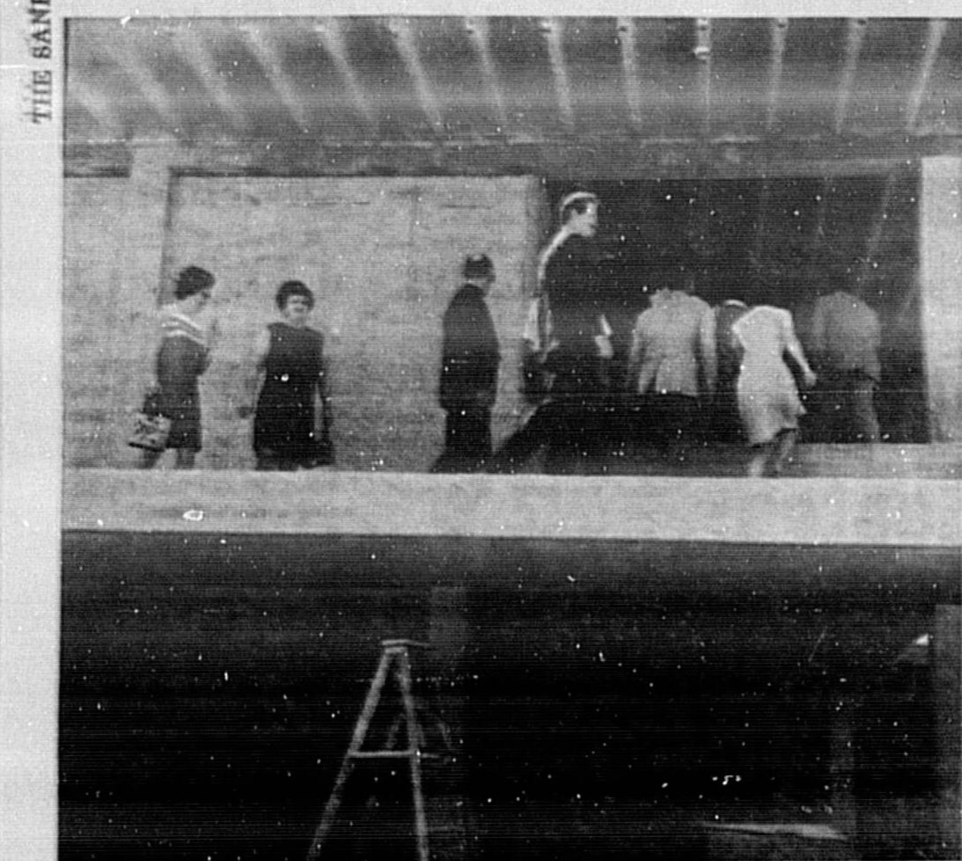
TOURING the new facilities under construction at Seminole Junior College were 42 high school counselors from Seminole and Orange counties as part of the third annual Counselor Orientation Day with Director of Administrative Affairs R. T. Milwee serving as guide. (Melinda Casselberry Photo)
