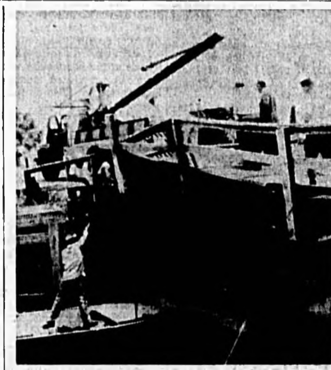
Scene Of The Repair Job
