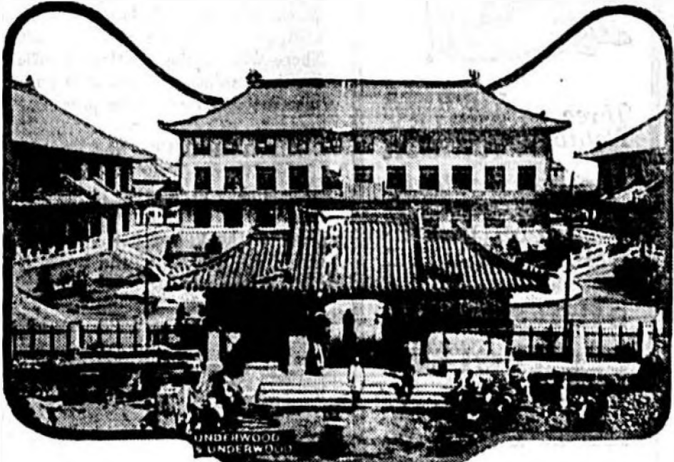
A view of the entrance court of the Peking Union Medical college, just opened and dedicated.
