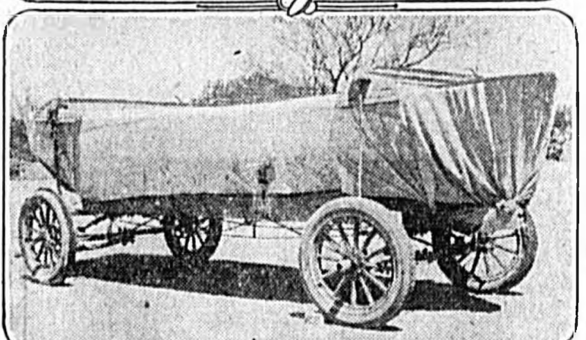
Before Harold Bell Wright entered the ministry and began writing novels he was a carpenter. Being also a fisherman and having his estate near Tucson, Ariz., a long way from the water, Wright designed and built the water diver shown above. He uses an outboard motor when chasing the finches, and he chases them all over. He takes the boat with him wherever he goes, and first launched it in the Gulf of California.
