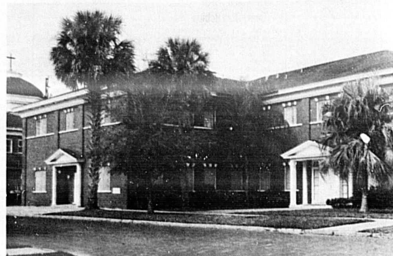
THE FIRST METHODIST CHURCH OF SANFORD ADDED ITS EDUCATIONAL BUILDING ON MAGNOLIA AVENUE AT FIFTH STREET
