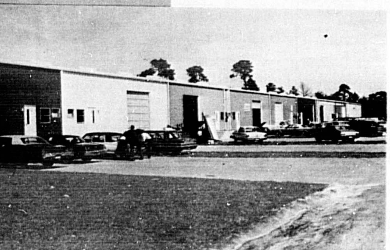
THIS IS THE EXISTING SPAULDING WAREHOUSE. ANOTHER IS UNDER CONSTRUCTION.
