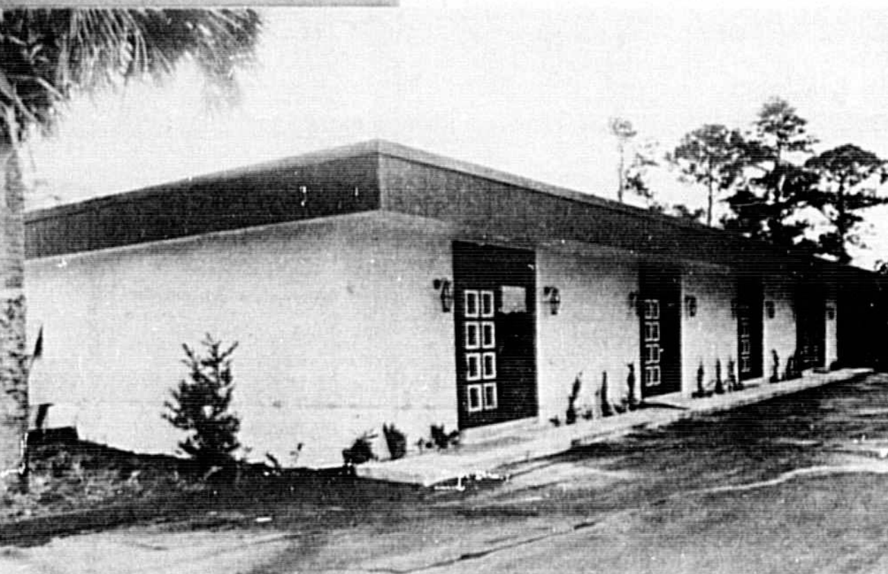
THE RECENTLY COMPLETED MEYER BUILDING IS ON FRENCH AVENUE AND 22nd STREET.
