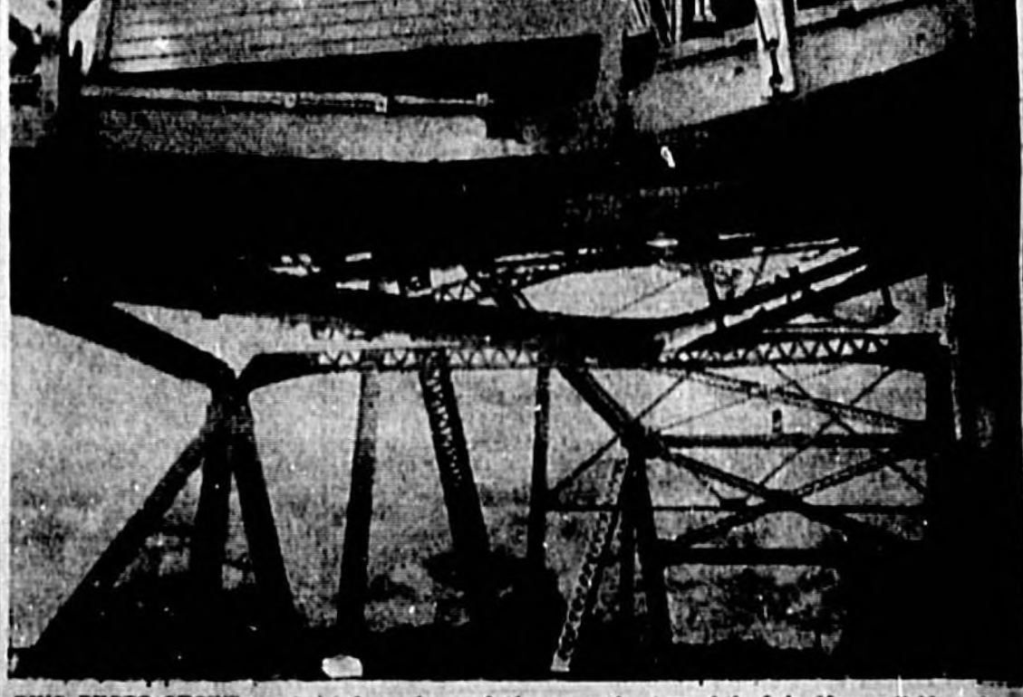
THIS PHOTO SHOWS the twisted wreckage of the upper structure of the Lake Monroe Bridge after a heavily loaded truck with cargo too high to clear the bridge tore into the steel and wood. Note the two steel beams, one bent outward and the other inward, caused by the bouncing of the cargo when it fell. (Staff Photo)
