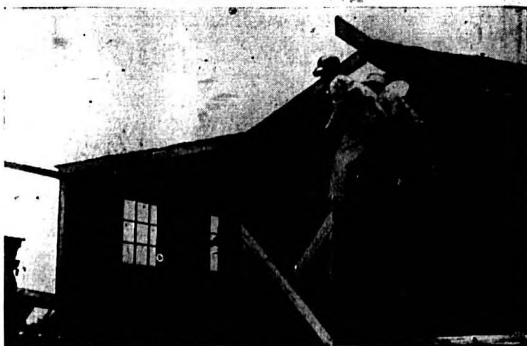
NO FOOD WAS SERVED in above mess hall being dismantled with rest of $20,000 CCC camp near Odesa, Del. Camp, built in 1925 for mosquito control program, wasn't used.
