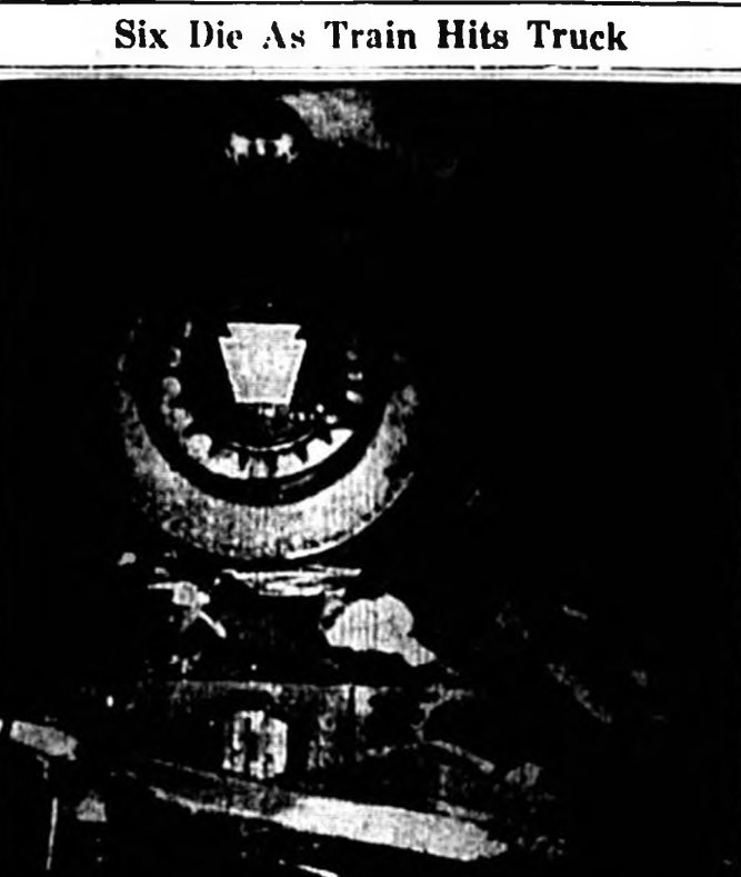
Six men were instantly killed and a seventh critically injured at Mincola, L. I., when the Fairbank, crack express train, hit a truck carrying the workmen from their jobs. Shown is a view of the truck's wreckage as it impaled on the locomotive.
