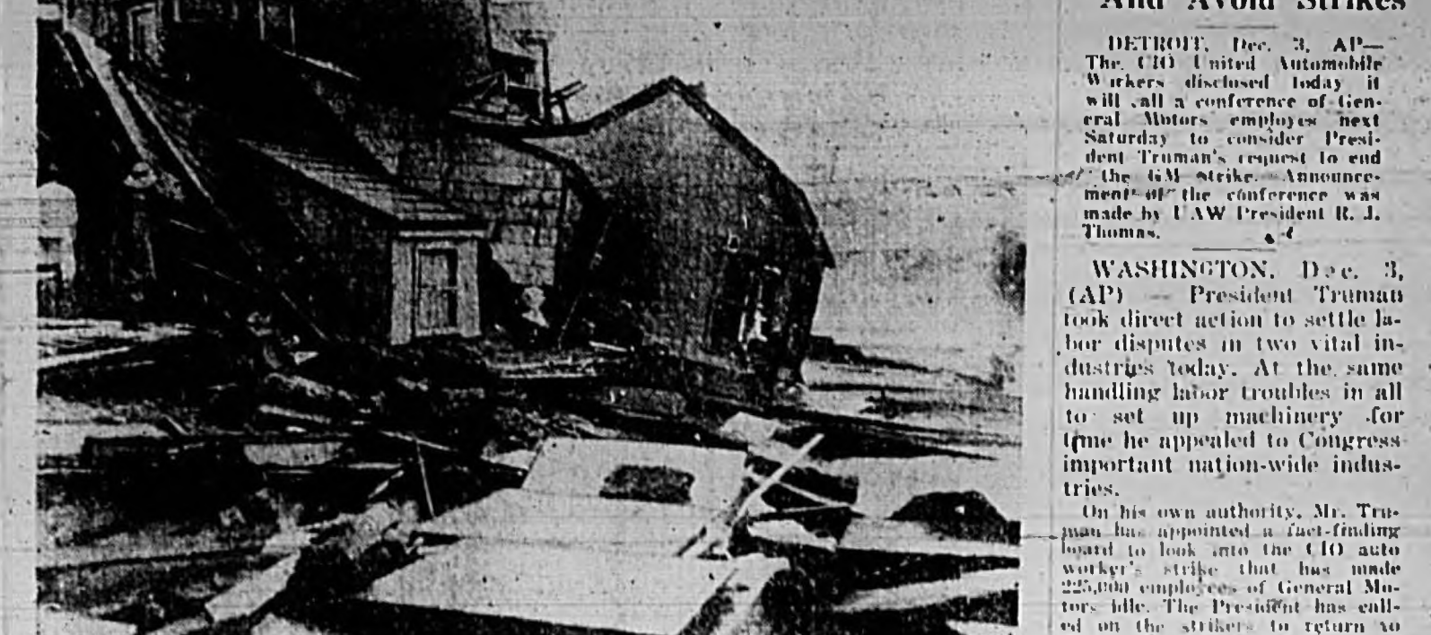
TUMBLING INTO THE ROUGH SURF as though they were made of paper mache, these houses in Winthrop, Mass., emphatically illustrate the fury of the Northeastern typhoon that lashed the coast. The great concrete slabs in the foreground were torn up by the roaring waters and tossed back like driftwood. The storm left in its wake at least thirty-four dead, numerous injured, and considerable property damage. (International Soundphoto)
