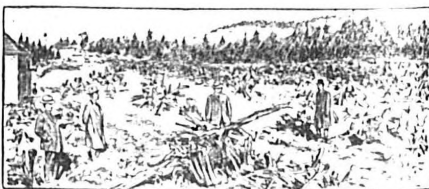
Drawn from actual photograph. Stumps blasted out into the ground.
