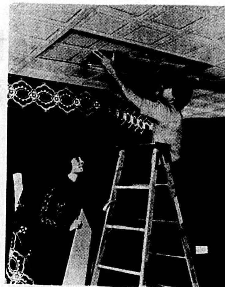
Young couples priced out of the new-home market are buying older homes and fixing them up themselves. A good place to start interior remodeling is at the top, with the ceiling, which is suspended below an old ceiling to hide cracking plaster or peeling paint.
