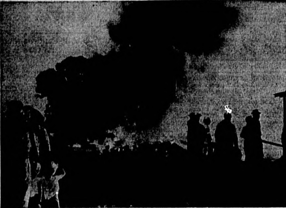
THREE HOMES were totally destroyed and a fourth damaged beyond repair by fire late Saturday on Sikes Ave. in the Midway section. The Navy Fire Dept., with later assistance from the Lake Mary Volunteer Dept., was credited with saving an additional three houses and a store along the row of buildings. (Herald Photo)
