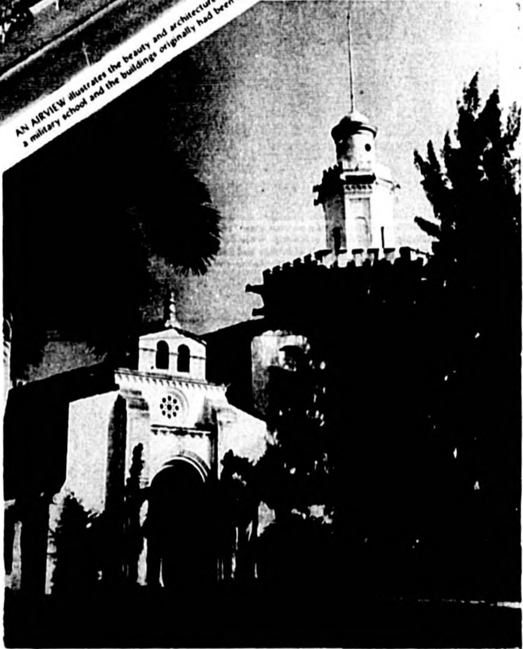
THE MAIN tower of Stetson's new College of Law (below) was copied from the famed Torre del Oro (tower of gold) in Seville.
