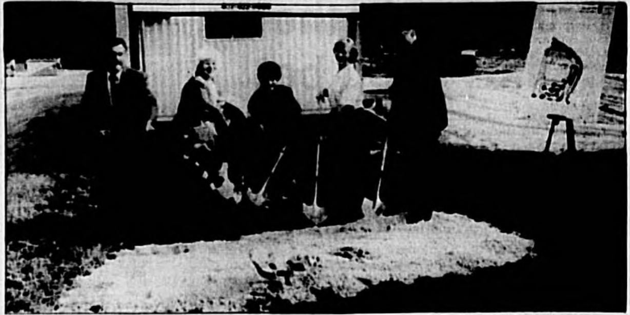
School board members break ground on a new district building project.
