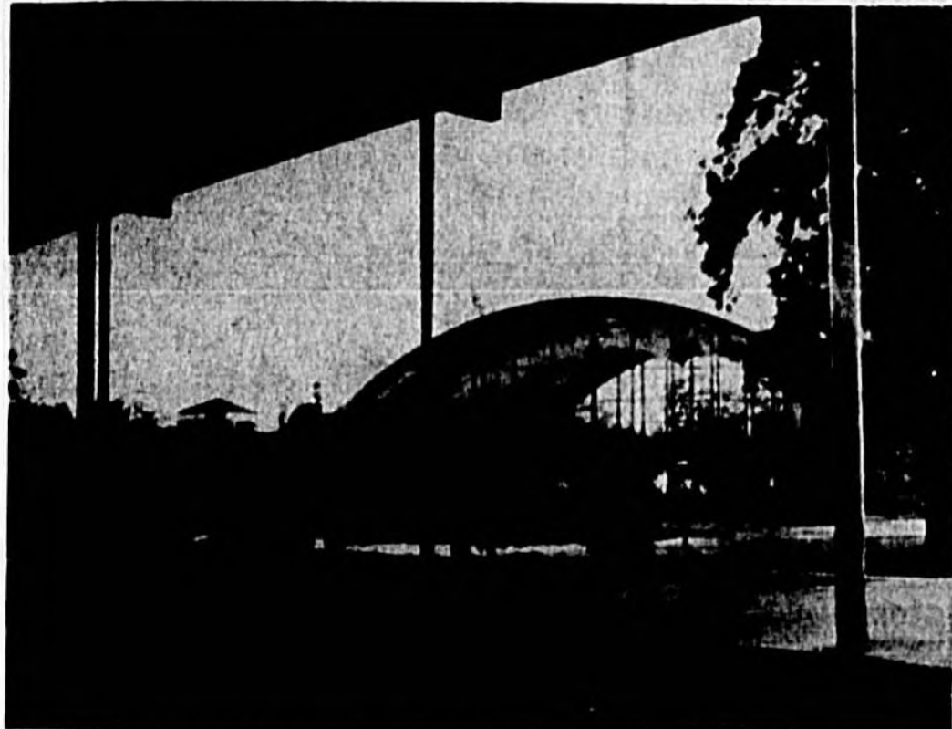
ARTISTRY in steel, glass and concrete form the graceful flowing lines of the beautiful Sanford Civic Center. The truly outstanding piece of modern architecture is the hub of Sanford's entertainment and social activities throughout the year.
