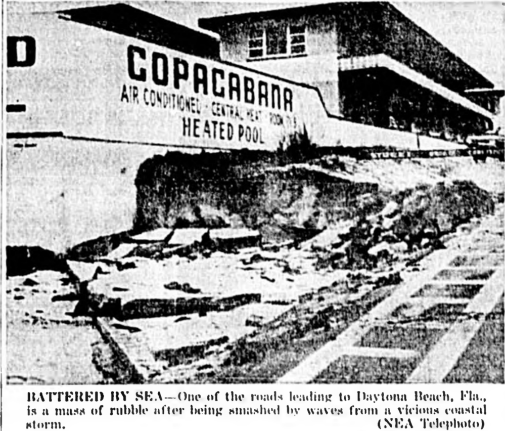
BATTERED BY SEA—One of the roads leading to Daytona Beach, Fla., is a mass of rubble after being smashed by waves from a vicious coastal storm.
