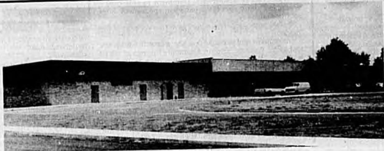
New Keeth Elementary School...getting finishing touches
