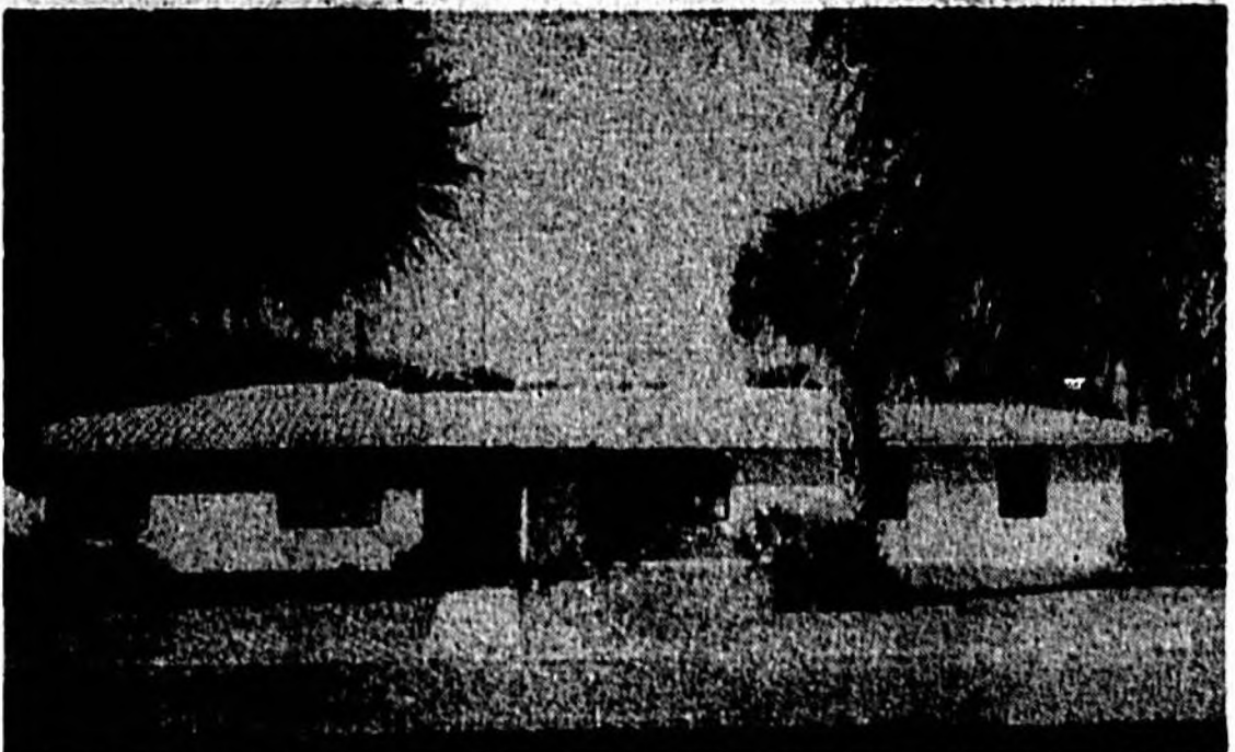
W. R. WILLIS of the Mayfair section of Sanford is the owner of the spacious home above. It was constructed by Ozier-Weller Homes, Inc. and consists of three bedrooms, bath, kitchen, and living room. A custom built home, it was especially designed for comfortable living in tropical areas.
