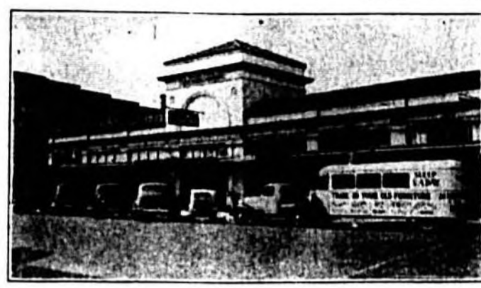
The McLander Avenue Building, recently acquired by the partner Furniture Co., which occupies a large portion of the structure has been completed to house and display the products sold by this widely known concern.
