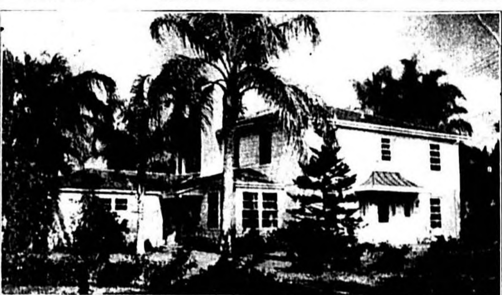
Among the most beautiful homes of Central Florida recently completed is that of Edmund B. Stowe, located at Indian Mound Village, overlooking the St. John's River. The residence is of partial masonry and frame construction with a single tile roof. It is insulated with rock wool and concrete and terrazzo floor, lined with a copper termite shield, insulating against the ravages of termites and the attacks of insects.
